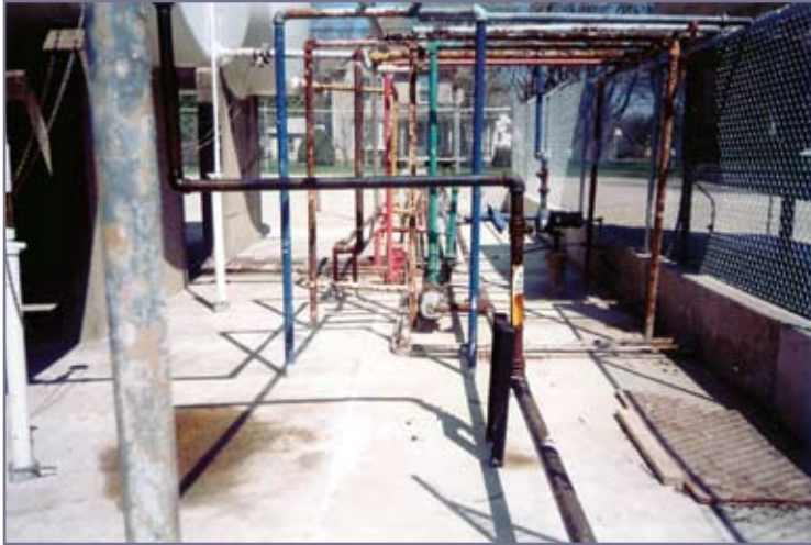
View of secondary containment and compliance with zero business interruptions to our client.
